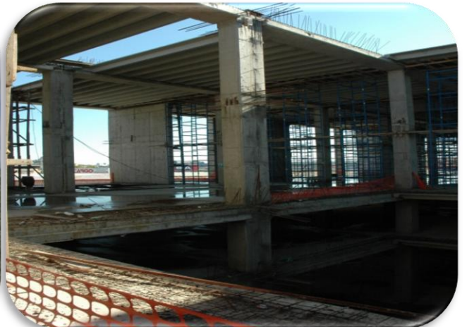
Prefabricated Building Shopping Mall – Gebze / TURKEY
