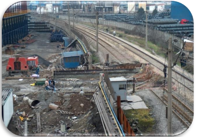
Prefabricated Slabs for Railway underpass / TURKEY
