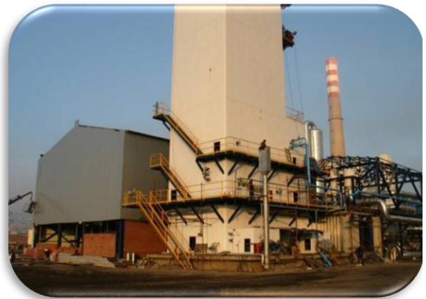
Cooling Tower – GEBZE/TURKEY
