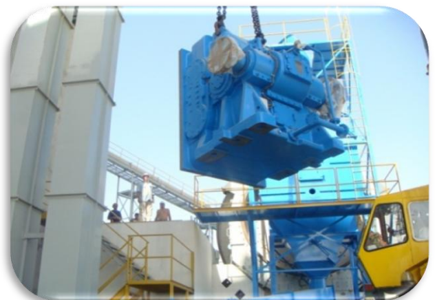
Cement Grinding Plant Construction Stages - UAE
