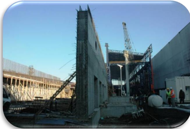
Steel Mill Structures – DİLOVASI /TURKEY
