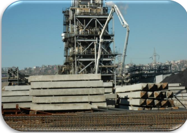
Precast Concrete Piles - Gebze / TURKEY
