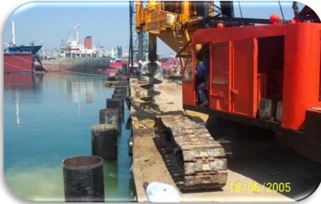
Jetty Piling Works- ISTANBUL/TURKEY
