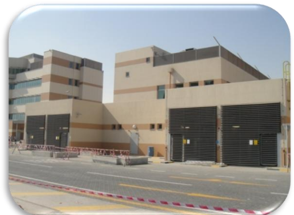
Berth 7 Substation Building STFA/QP – DOHA/QATAR
