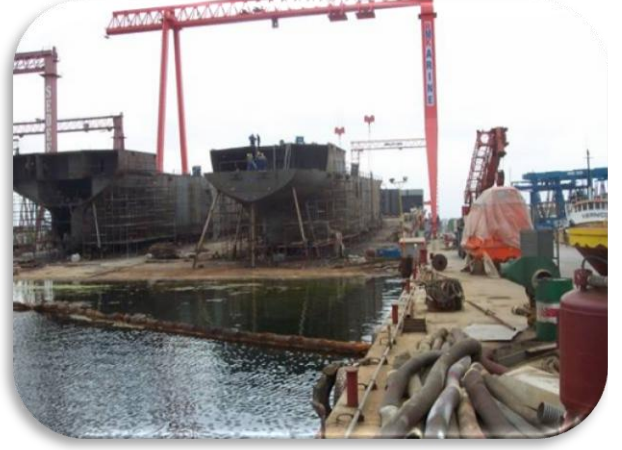
Marine Works – RMK TUZLA/TURKEY
