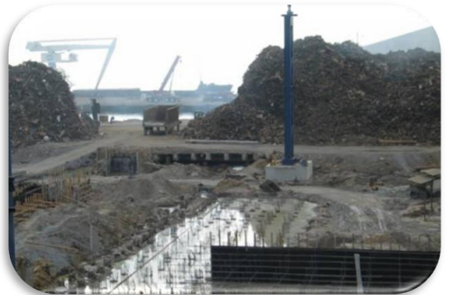
Soil Improvement at Steel Plant – DİLOVASI/TURKEY
