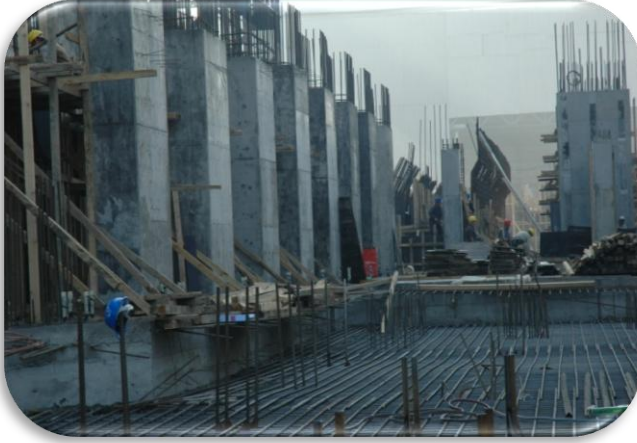
Steel Plant Structures - DİLOVASI/TURKEY
