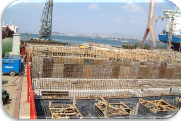
Shipyard Construction – TUZLA/TURKEY
