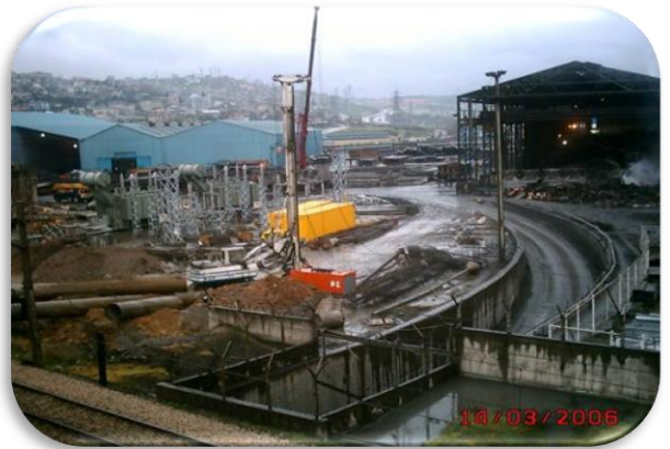
Pile Works for under ground railway pass
