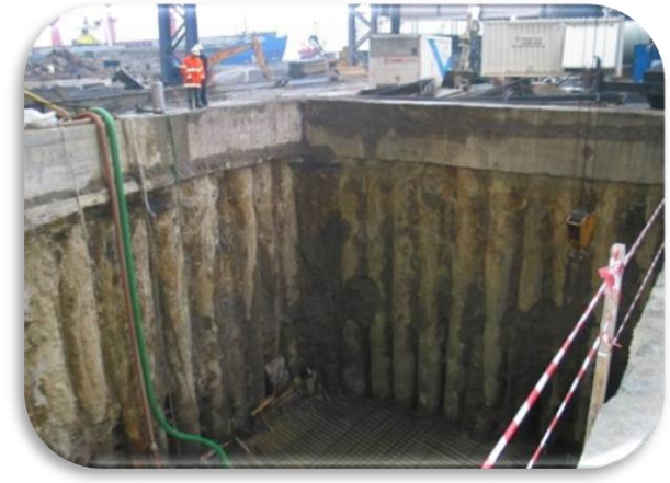
Caisson Works – DİLOVASI/TURKEY
