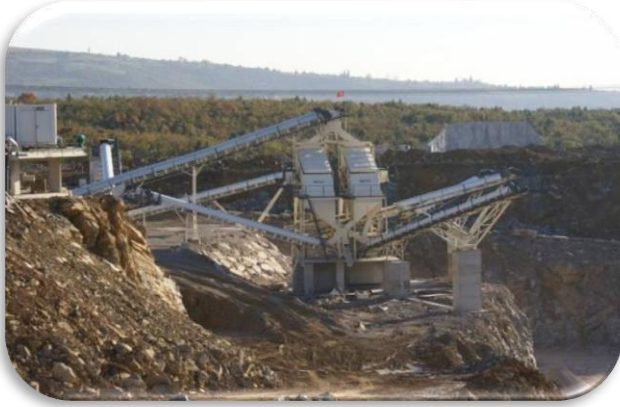
Quarry Plant – GEBZE/TURKEY
