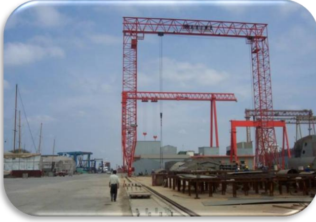
Slipway Construction – RMK TUZLA/TURKEY
