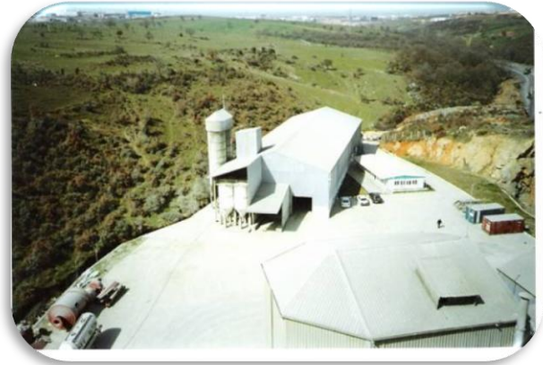
Construction Chemicals Plant – GEBZE/TURKEY
