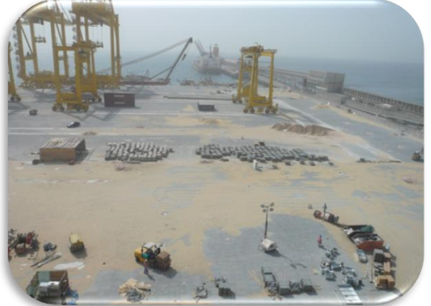
Berth 7 Paving works STFA/QP – DOHA/QATAR
