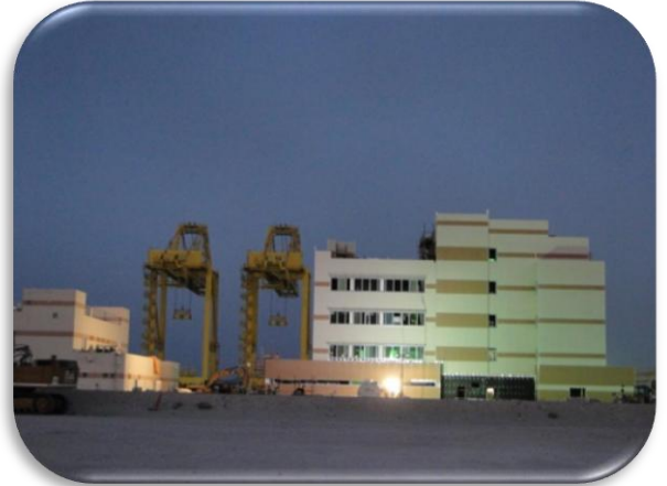
Berth 7 Office Building STFA/QP – DOHA/QATAR
