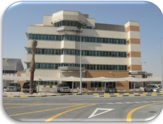
Berth 7 Office Building STFA/QP – DOHA/QATAR
