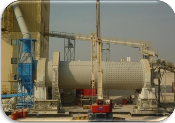
Cement Grinding Plant Construction Stages - UAE
