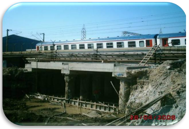
Under Railway Pass Construction – DİLOVASI/TURKEY
