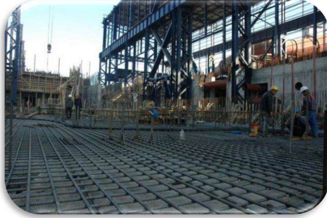
Steel Mill Structures – DİLOVASI /TURKEY
