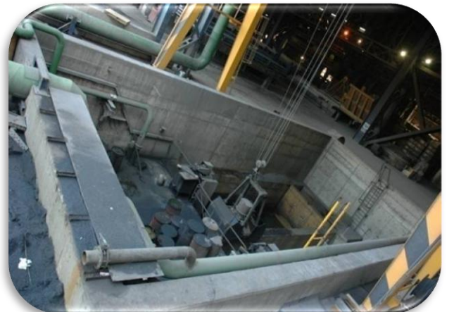
Caisson Works for Steel Plant – DİLOVASI/TURKEY
