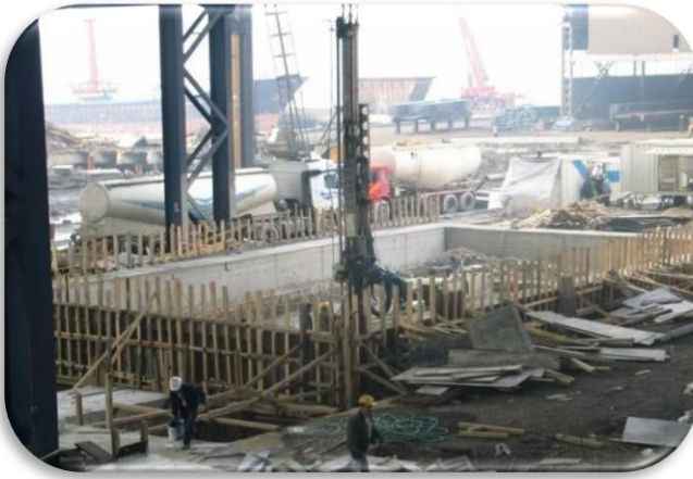
Caisson Works – DİLOVASI/TURKEY
