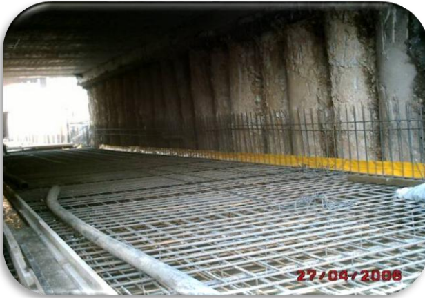
Under Railway Pass Construction – DİLOVASI/TURKEY
