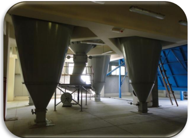
Cement Grinding Plant Construction Stages - UAE
