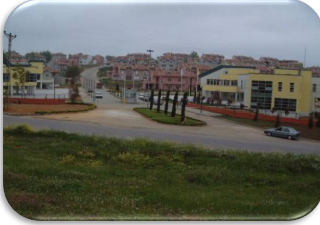
Infrastructures of Housing Complex – ISTANBUL/TURKEY
