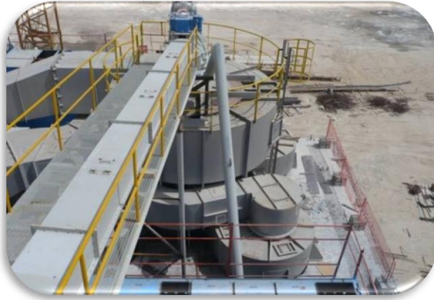
Cement Plant Installations – UAE
