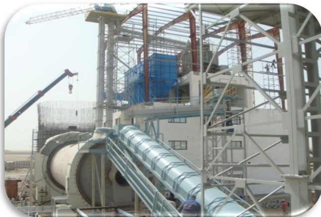
Cement Grinding Plant Construction Stages - UAE
