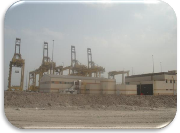
Berth 7 Substation Building STFA/QP – DOHA/QATAR
