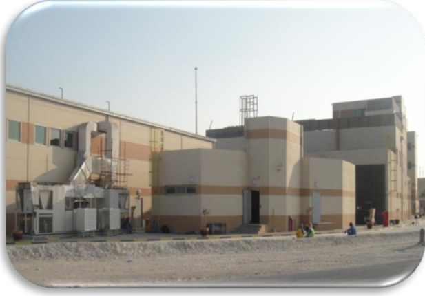
Berth 7 Substation Building STFA/QP – DOHA/QATAR
