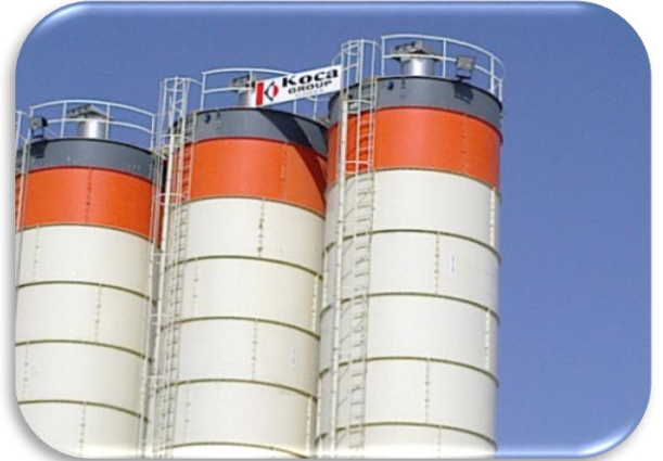
Ready Mix Concrete Plant – RIYADH/KSA
