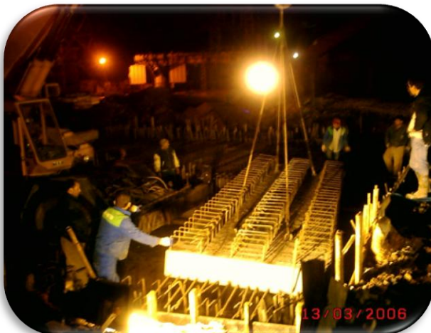
Installations of Prefabricated Elements - TURKEY
