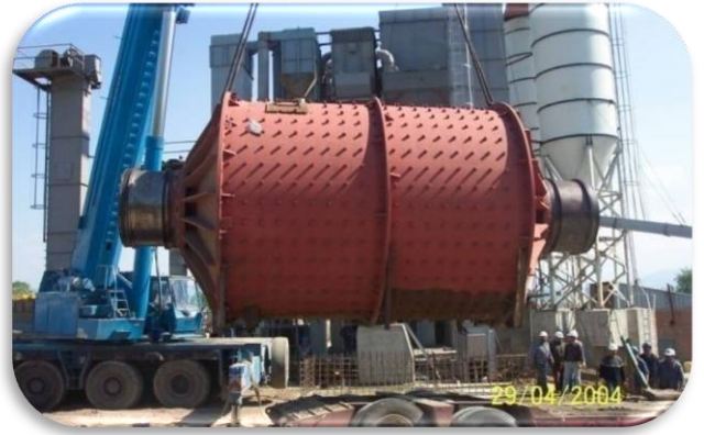
Installation of Grinding Mill – ÇAN/TURKEY
