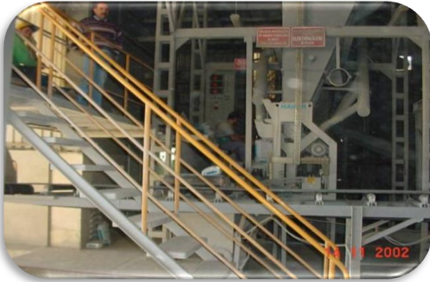
Construction Chemicals Plant – GEBZE/TURKEY
