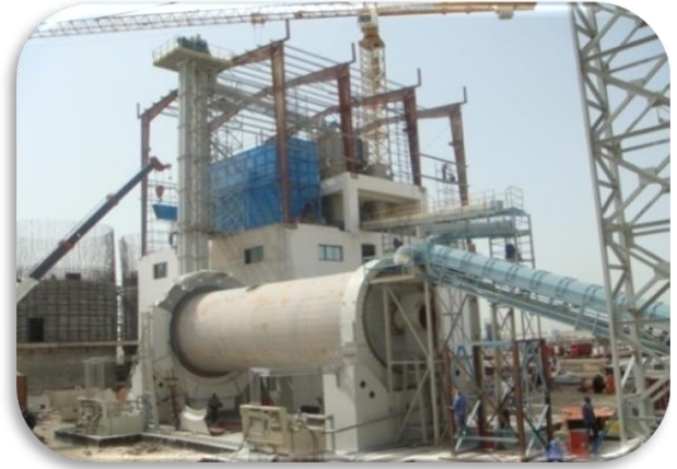
Completion of Cement Plant – UAE
