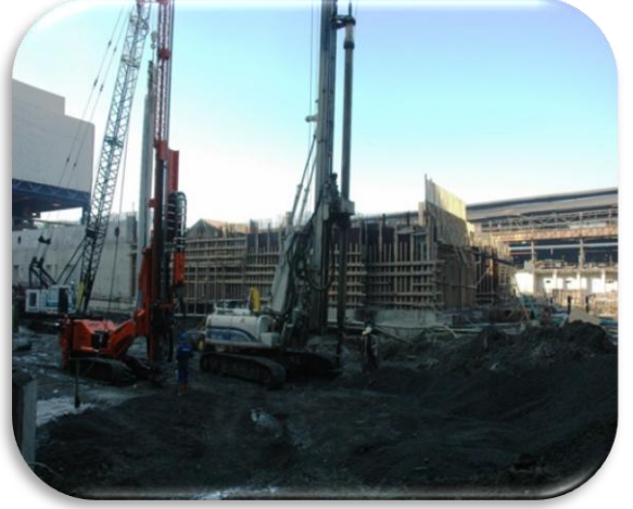
Soil improvement works
