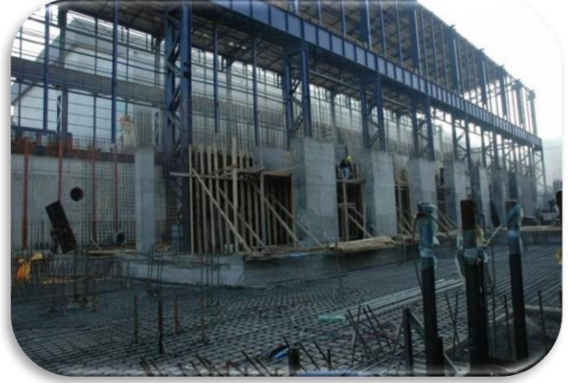
Steel Mill Structures – DİLOVASI /TURKEY
