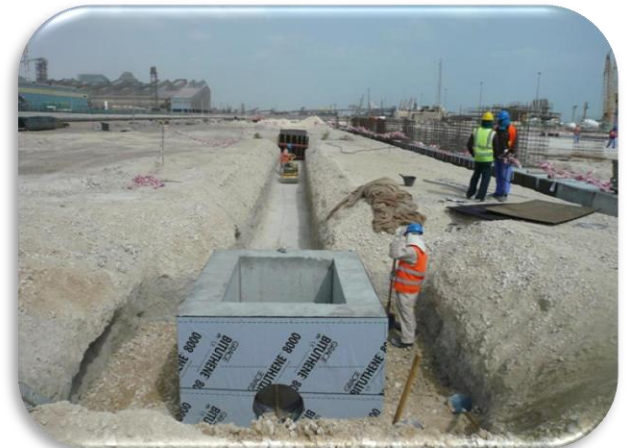
Prefabricated Manhole and trenches - Doha / QATAR
