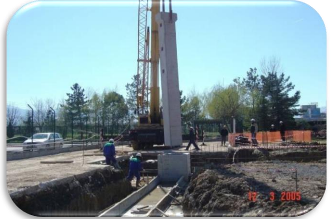
Precast elements building a factory – KOCAELI/TURKEY
