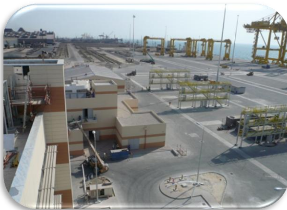
Berth 7 Paving works STFA/QP – DOHA/QATAR
