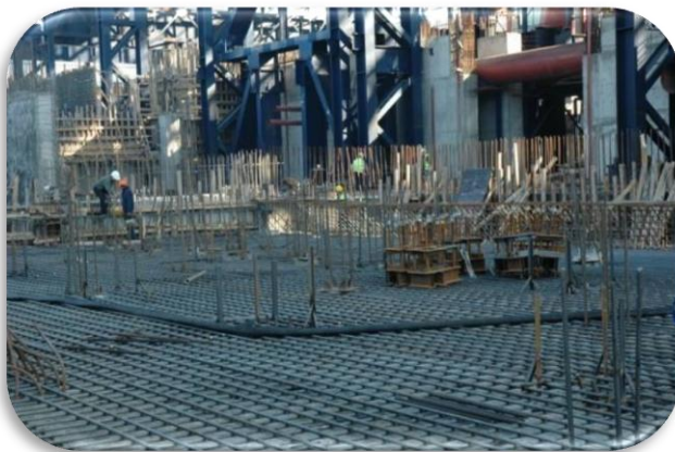
Steel Plant Foundation Structures – DİLOVASI/TURKEY
