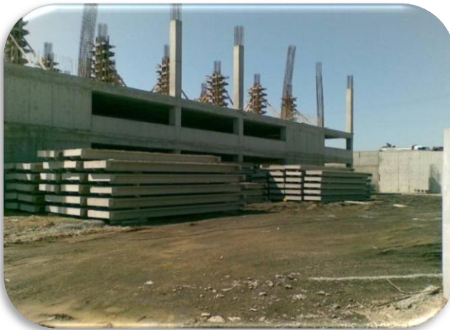
Precast Slabs for a Mall – TURKEY
