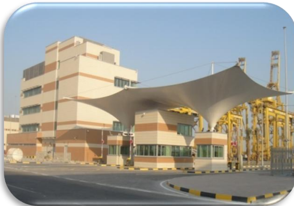
Berth 7 Office Building STFA/QP – DOHA/QATAR
