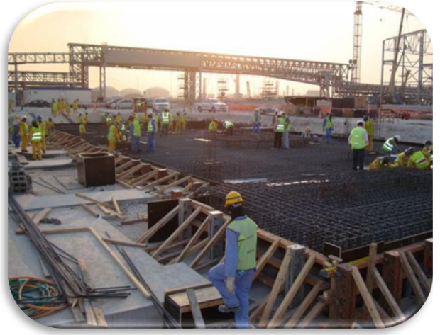
Berth 7 Office Building STFA/QP – DOHA/QATAR
