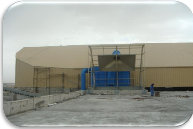
Completion of Cement Plant – UAE
