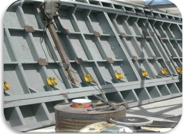
Harbor Repairing Works – LIBYA
