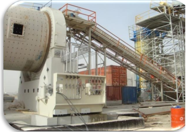
Cement Grinding Plant Construction Stages – UAE
