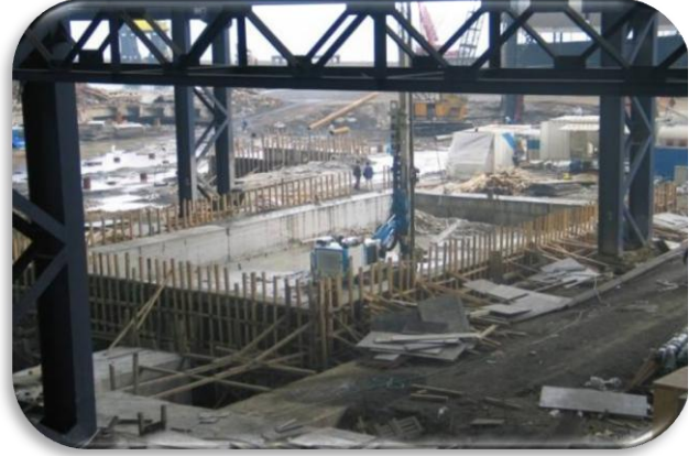
Caissons Construction – DİLOVASI/TURKEY
