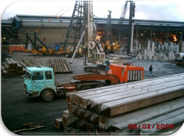
Prefabricated Piles – Steel Plant / TURKEY
