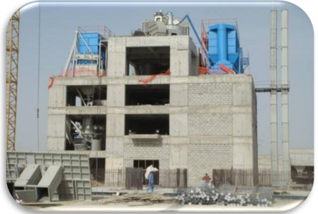
Cement Plant Installations - UAE
