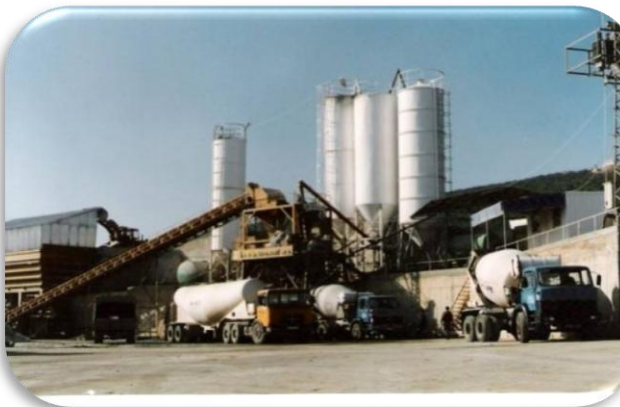
Ready Mix Concrete Production – GEBZE/TURKEY
