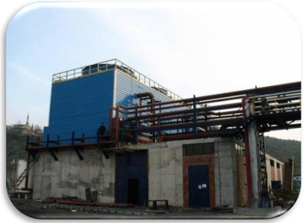
Power Generating Structures – DILOVASI /TURKEY
