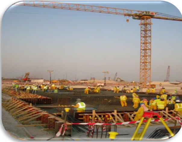
Berth 7 Office Building STFA/QP – DOHA/QATAR
