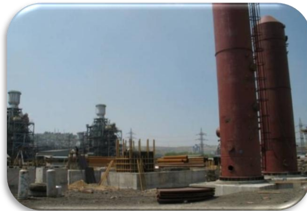
Steel Plant Structures – DİLOVASI /TURKEY
