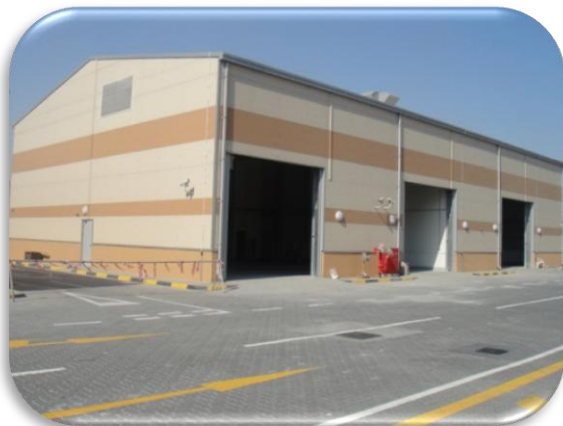
Berth 7 Substation Building STFA/QP – DOHA/QATAR
