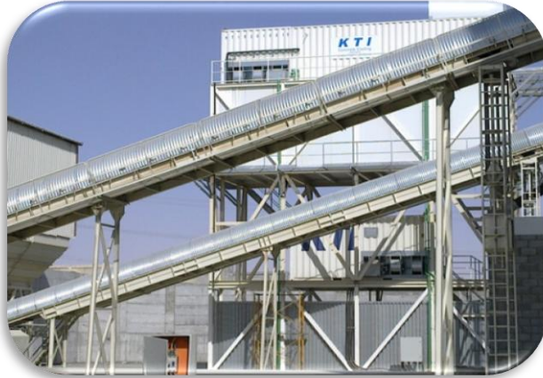
Ready Mix Concrete Plant – RIYADH/KSA
