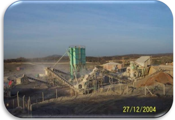
Quarry Plant– GEBZE/TURKEY
