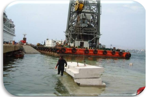
Pile Cap & Slabs Placement – TUZLA/TURKEY
