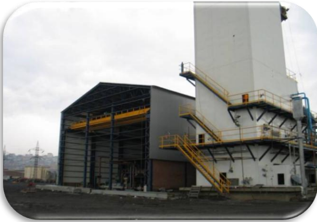
Cooling Tower – DILOVASI/TURKEY
