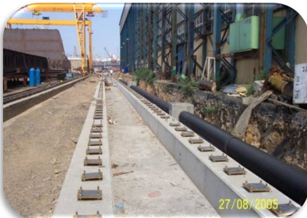
Crane railway construction – ISTANBUL/TURKEY
