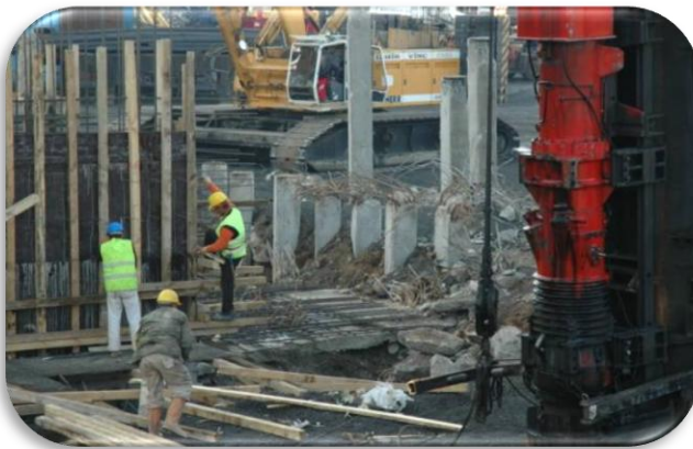
Various Pile Works - Foundations
