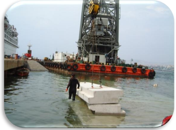
Construction of Shipbuilding Yard Slipway RMK Marina
