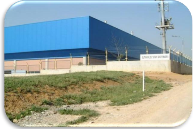
Metal Fabrication Factory – KOCAELI/TURKEY
