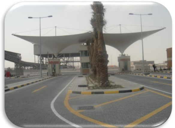
Berth 7 Office Building STFA/QP – DOHA/QATAR
