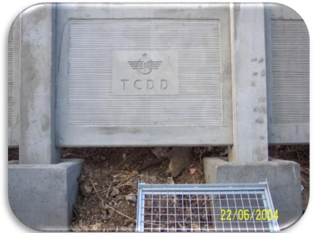
Precast Railway Walls - TURKEY
